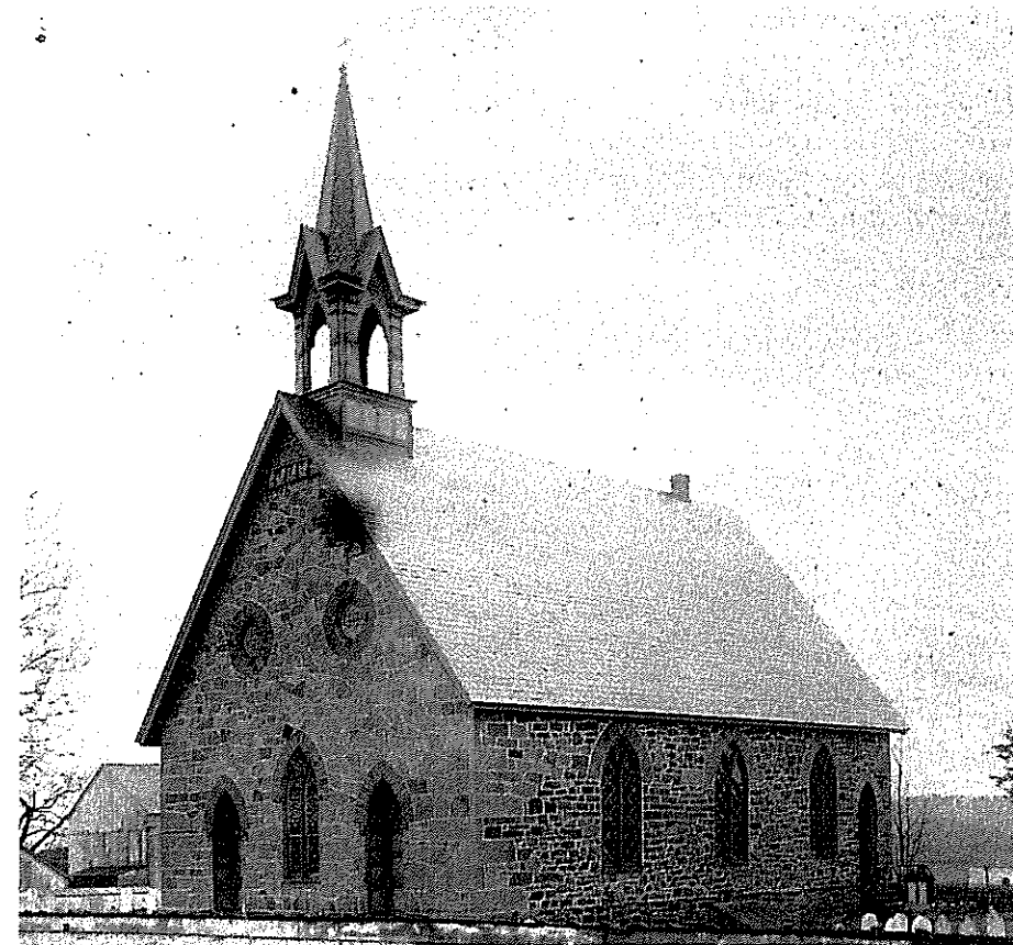
Bangor Episcopal Church, Churchtown, Caernarvon Township, c. 1885. This stone church, built in 1830, replaced another stone church built in 1754–56, which in turn replaced a log structure built in about 1733. At some time in the nineteenth century, the present church was remodeled with mid-Victorian features. Photo courtesy of the Episcopal Church of Bangor in Caernarvon.
